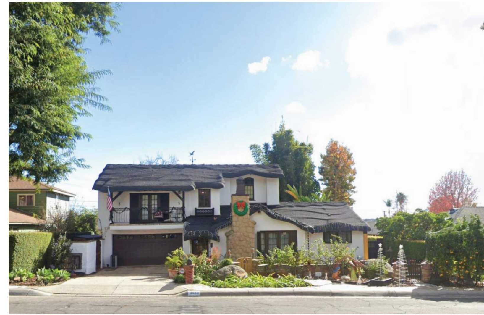
3043 PASEO DEL DESCANSO VIEW FROM STREET
