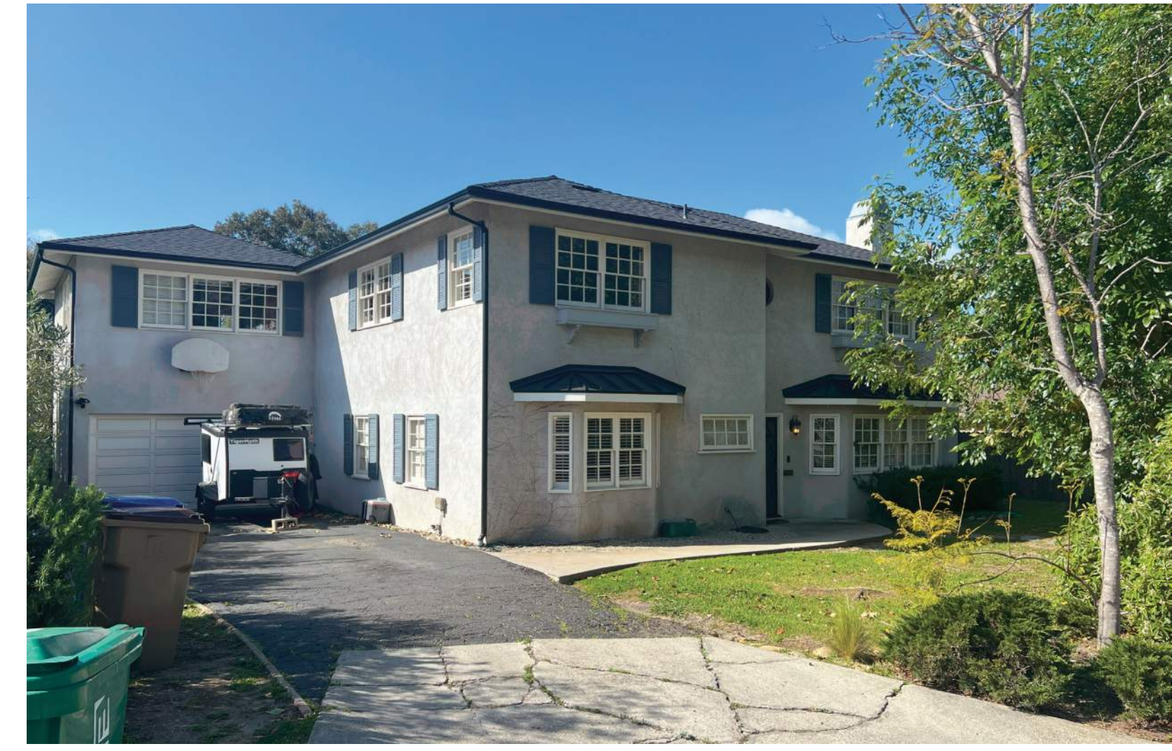
326 VISTA DE LA CUMBRE VIEW FROM STREET
