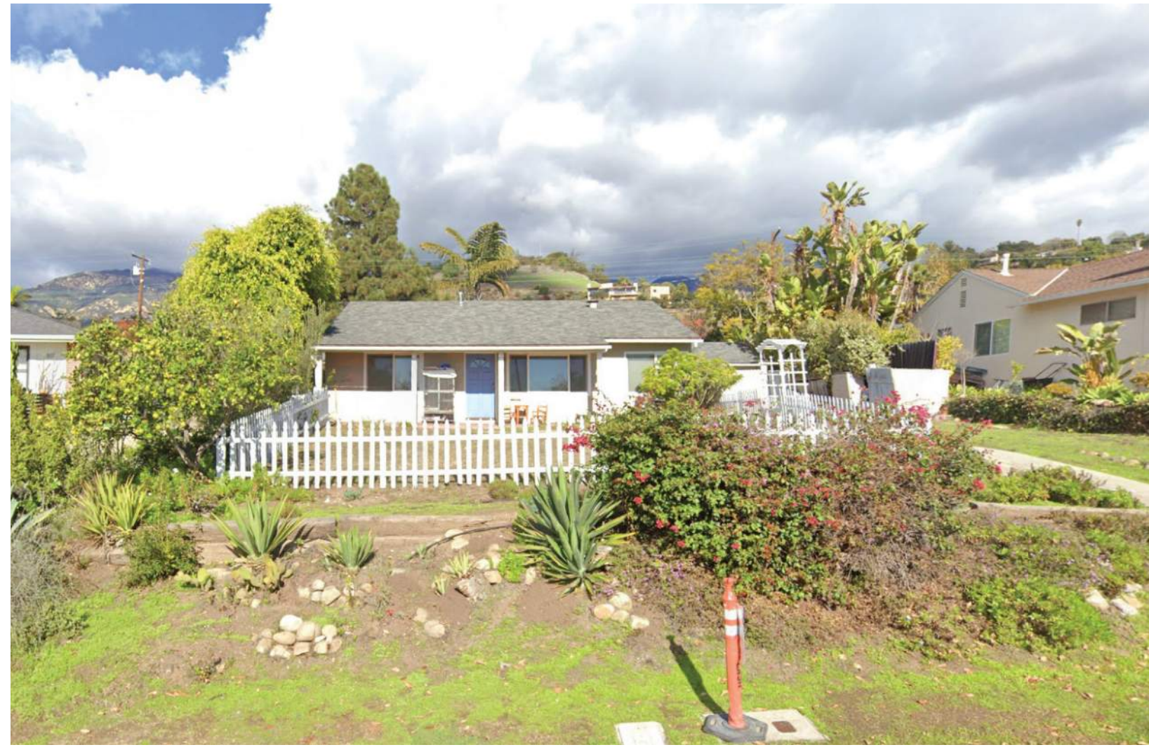
321 VISTA DE LA CUMBRE VIEW FROM STREET
