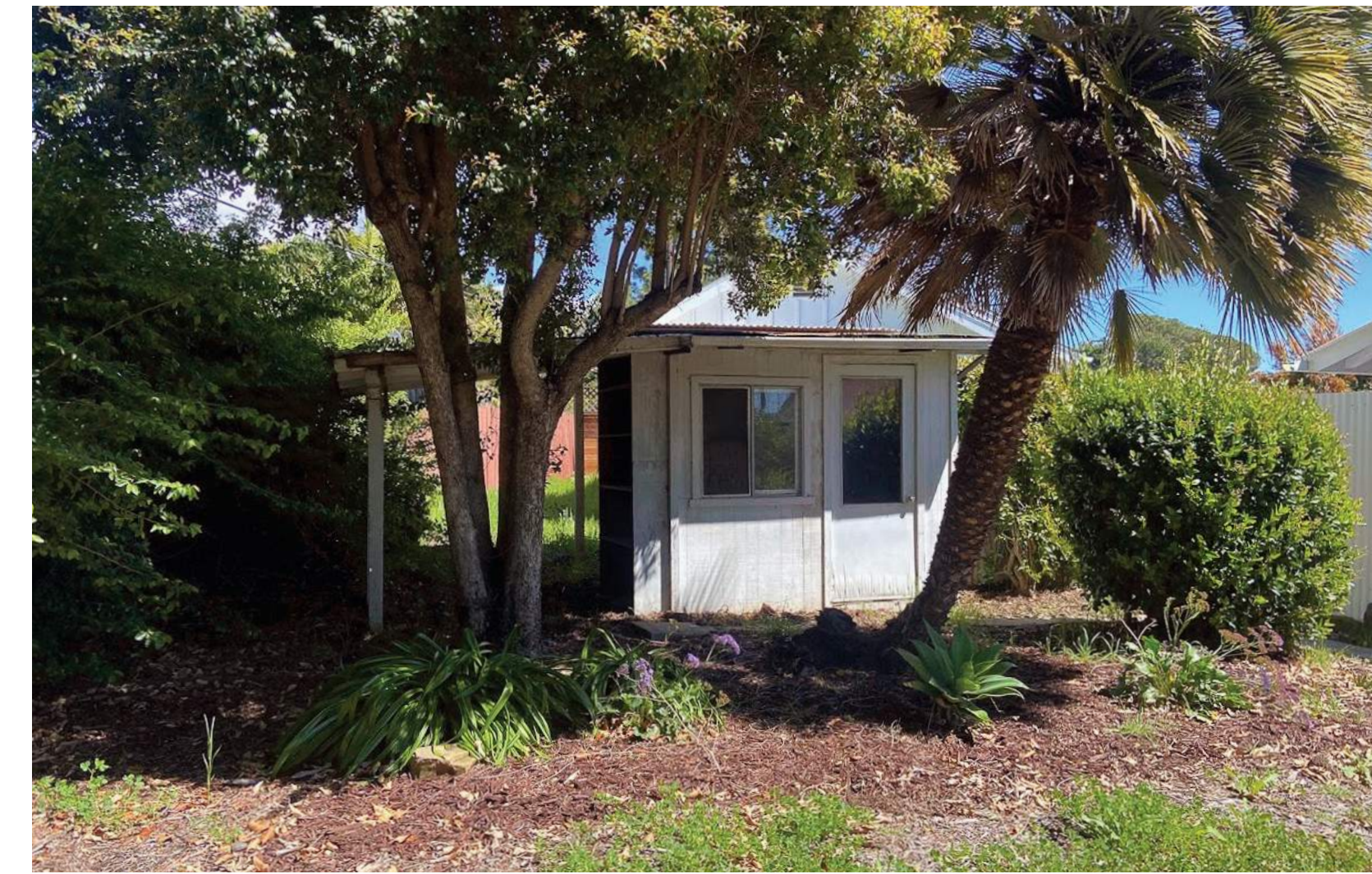
8: EXISTING WORKSHOP/SHED (TO BE DEMOLISHED)
