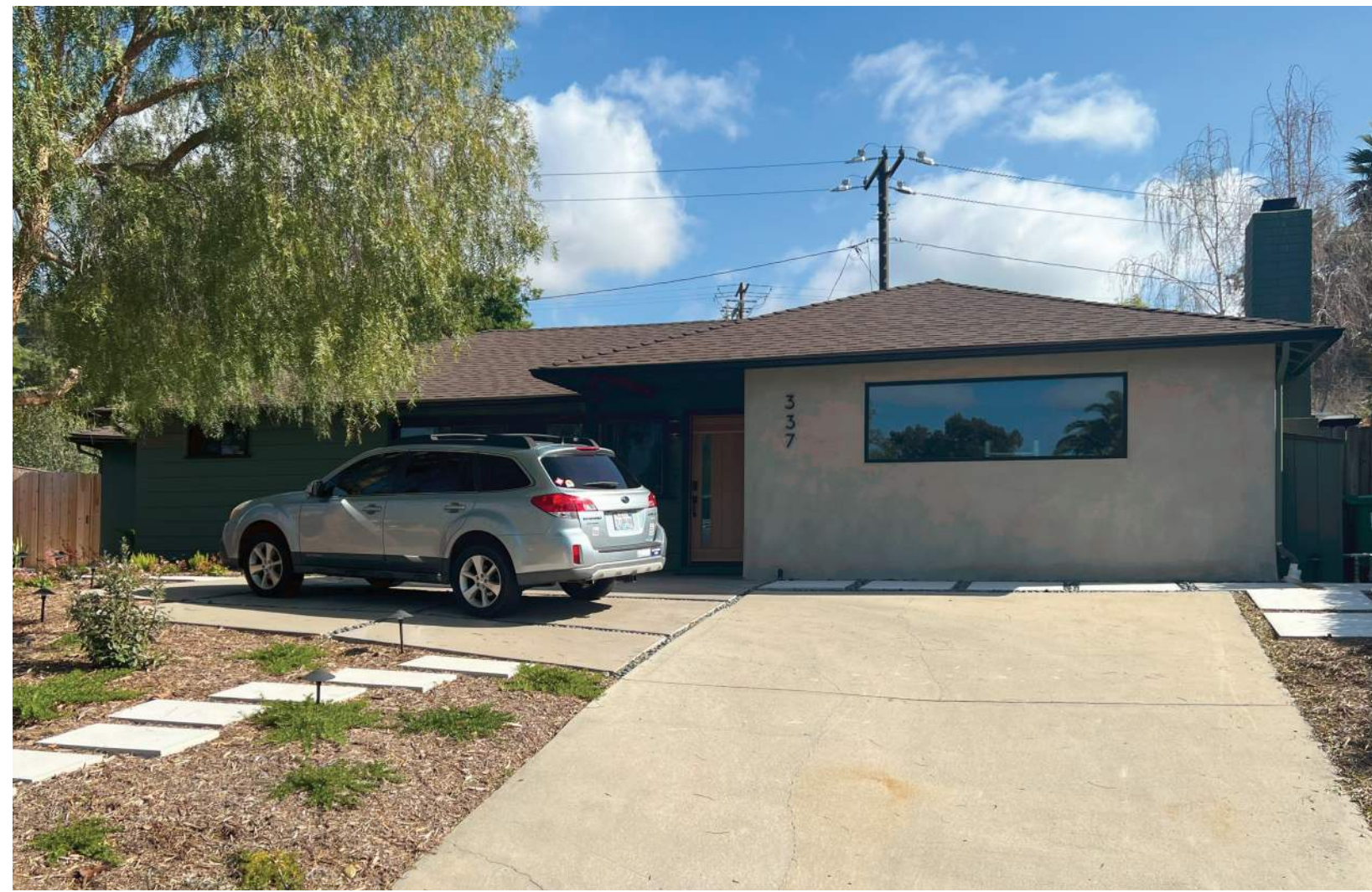
337 VISTA DE LA CUMBRE VIEW FROM STREET
