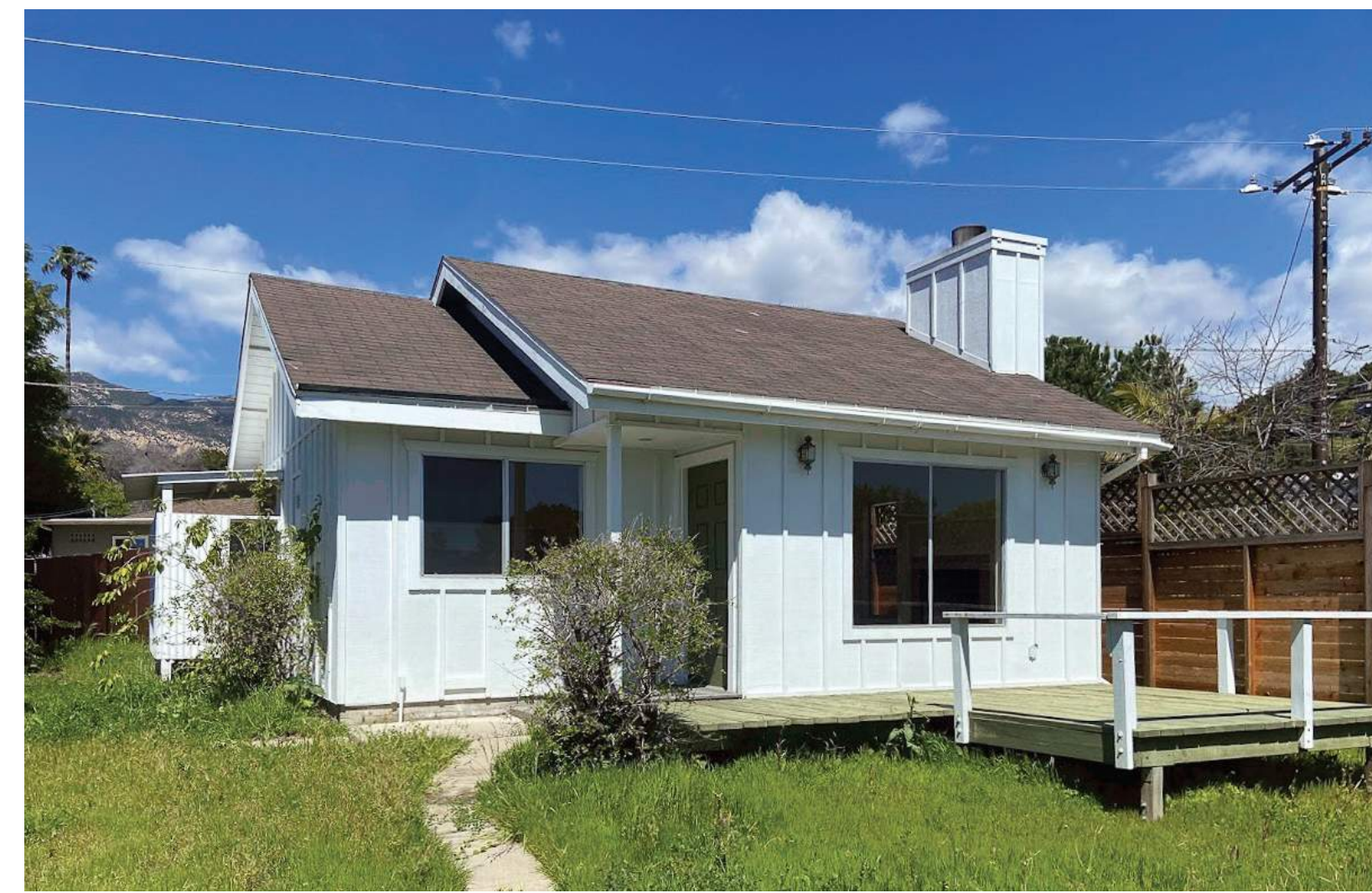
7: EXISTING ACCESSORY STUDIO (TO BE DEMOLISHED)
