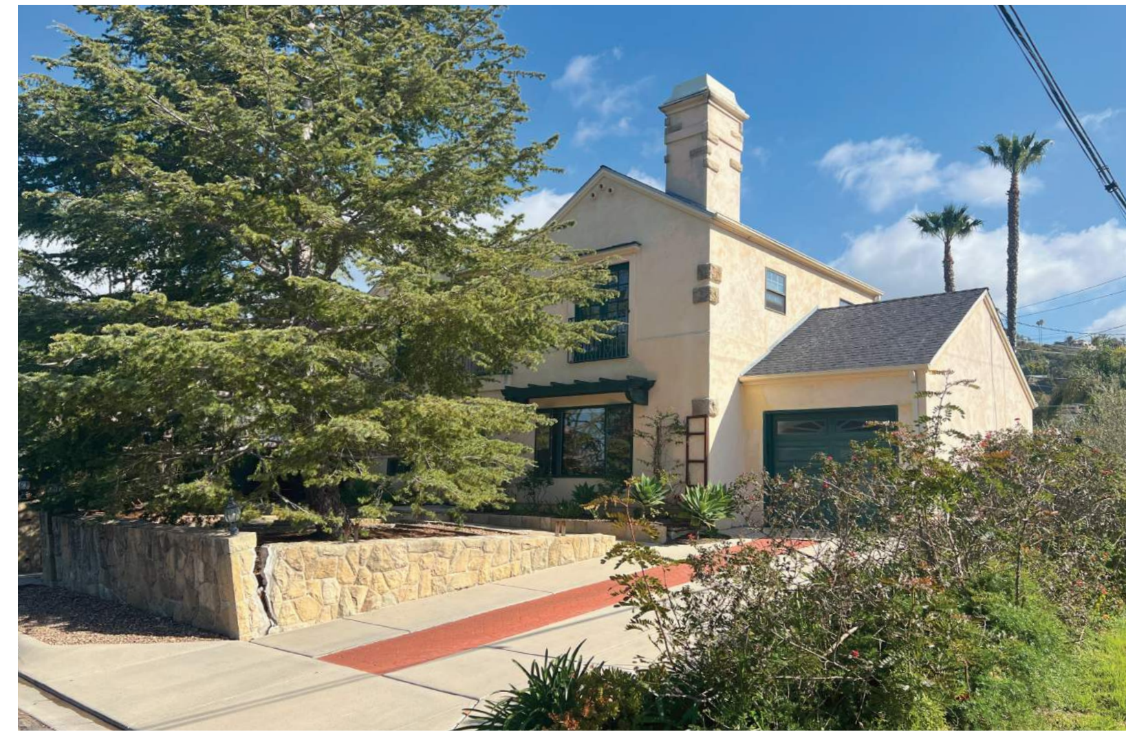
345 VISTA DE LA CUMBRE VIEW FROM STREET
